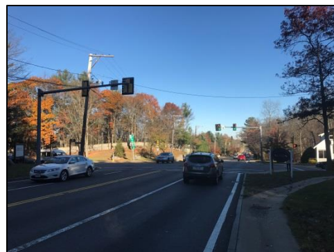
Lane use signage and pavement markings are not provided along the Route 28 northbound and southbound approaches.
